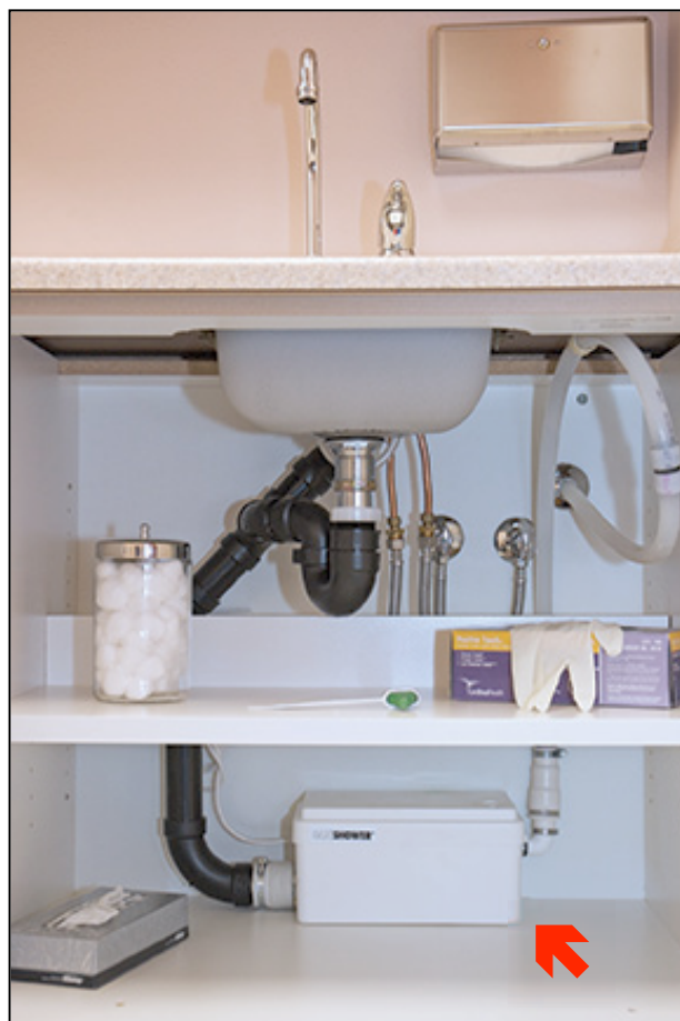
MEASURING ONLY 13 INCHES WIDE AND 6-1/2 INCHES DEEP, THE 6-INCH-TALL SANISHOWER UNIT (RED ARROW) IS SMALL ENOUGH TO FIT WITHIN A LAVATORY CABINET, LEAVING PLENTY OF ROOM FOR OTHER STORAGE.
