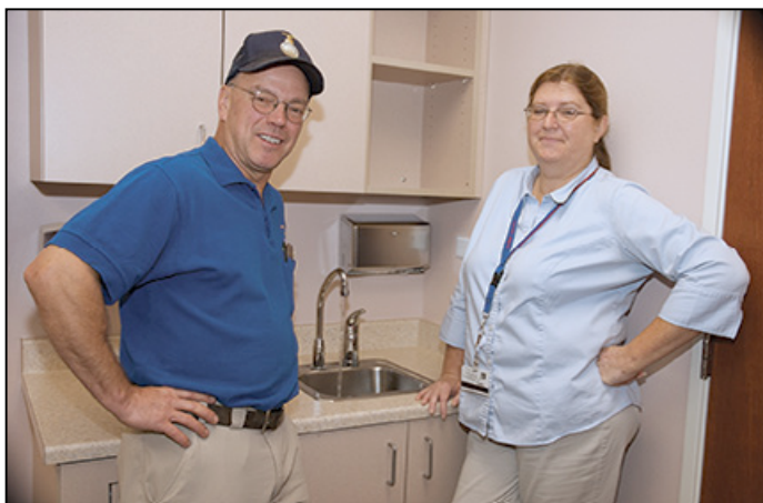
CONTRACTOR JOHN MORRIS AND KATHY SMITH, UKIAH VALLEY MEDICAL CENTER ADMINISTRATIVE DIRECTOR OF SUPPORT SERVICES, WITH ONE OF THE 22 SINKS THAT WERE FITTED WITH SANIFLO SANISHOWER GRAY WATER PUMPS (NOT SHOWN).
